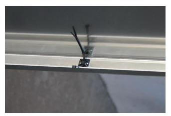
Thread one cable connector each through the latch of the self-adhesive cable brackets.
