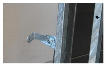
Mount the doors with the notch at the door stop pointing downwards.
